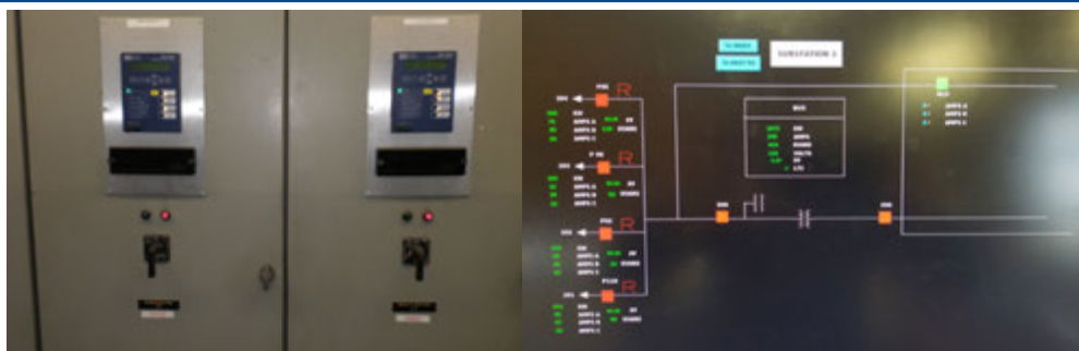
Pictured is one of the Village's substations with new smart relays installed on the substation breaker doors.
