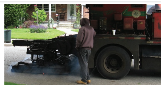
The "hot box" pothole repair machine.
